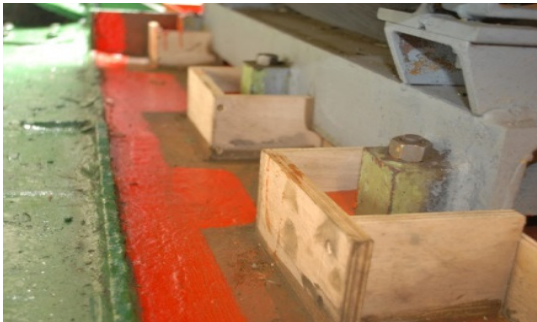
3. Product curing around bolts
