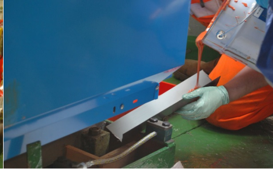
2. Pouring Belzona 7111 into the prepared area
