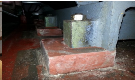
4. Completed application with dams removed
