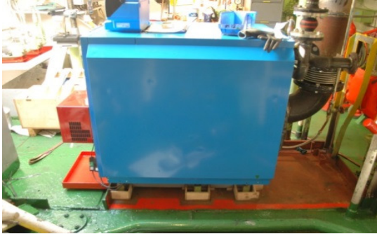
1. Boiler set in place
