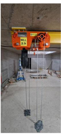
Offering a safe working load of 2.5t each, the hoists provide 8m of lifting height and run on beam lengths of 8.5m and 7.0m.
