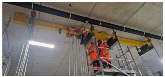
Once in position, the company proceeded with drilling operations and resin anchor installation for all ceiling anchor points after meticulously cleaning each hole with a special heavy-duty internal brush and suction pump.
