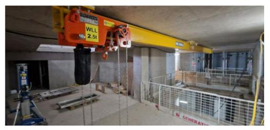
William Hacket low-headroom manual hoists were installed to overcome the issue of very tight headroom clearances due to the size of the equipment.
