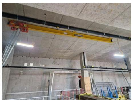
Hoist & Winch Ltd recently installed hoists for the successful lifting and transfer of a large energy plant within a residential tower block.
