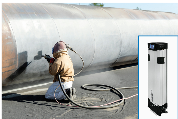
Breathing air supply for sandblasting work
