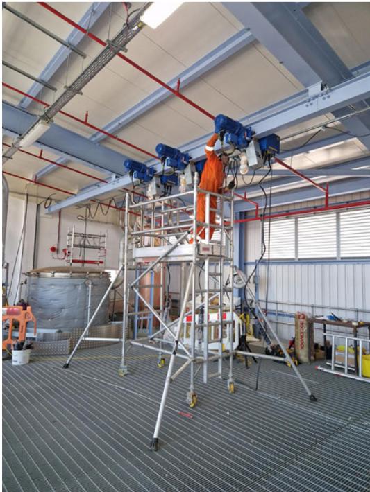
Among the challenges of this demanding project was a restriction in the overall height of the new building due to local planning laws.
