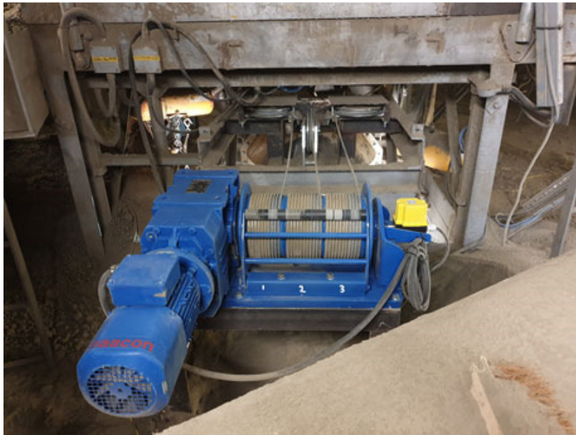
The bespoke electric winch used for the safe and smooth lifting and lowering of a large telescopic export chute.
