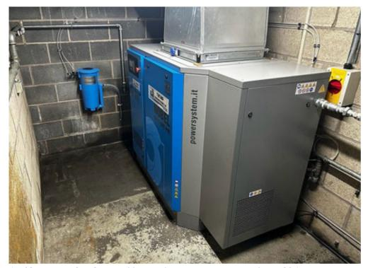
A NOBEL 18.508 DVF PM variable-speed screw air compressor from FPS Air Compressors systems has seen a 46% reduction in compressor energy consumption at Armac Martin.
