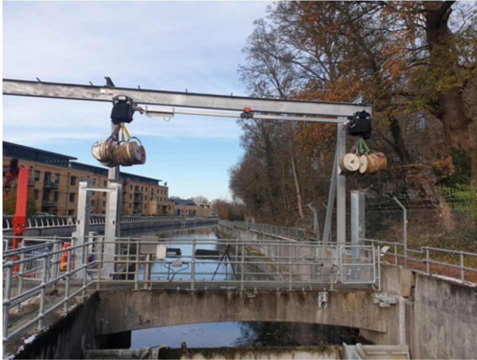
Tandem hoist rear view with test load.
