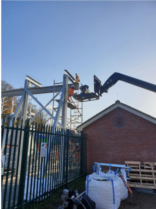
Tandem hoist installation - Telehandler & TEE Frame combination.
