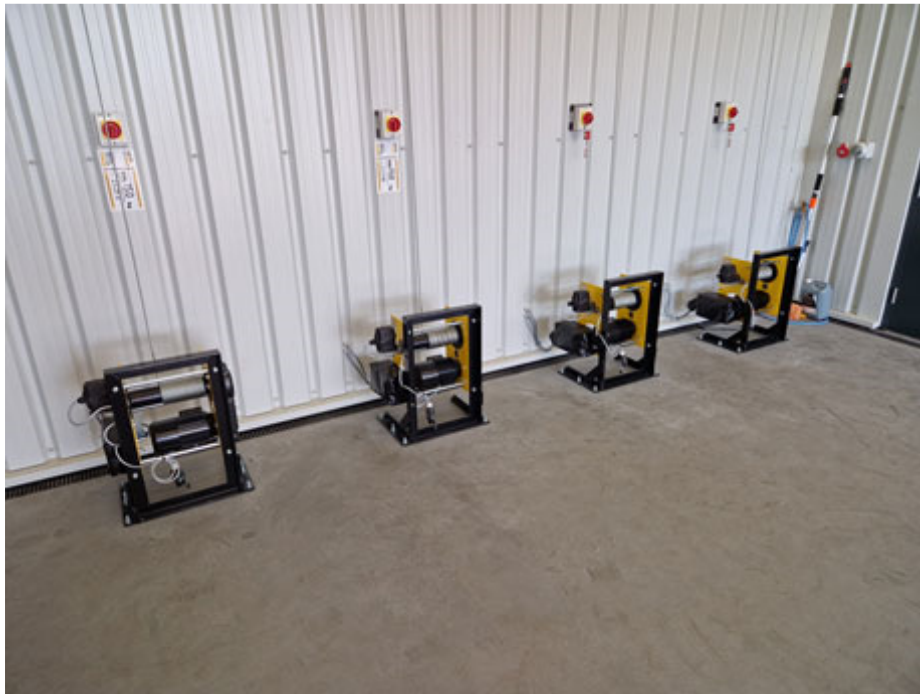
Winch installation in progress.
