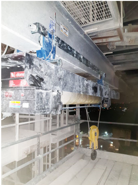
Wire-rope hoist in final position after installation and test by Hoist & Winch Ltd.
