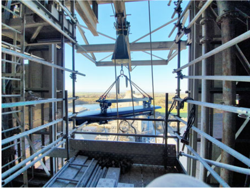
10-tonne SWL wire-rope hoist being lifted into position.
