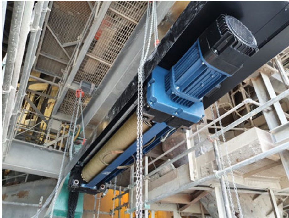
10-tonne SWL electric-powered wire-rope hoist unit lifted into final position at a 60m height by Hoist & Winch Ltd.
