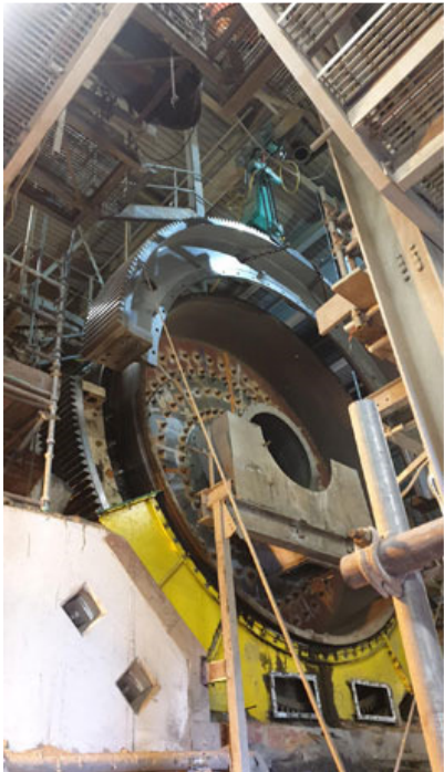
The hoist was necessary to spread the 9t load over a greater distance of the monorail beam bottom flange than a standard hoist trolley arrangement would allow.
