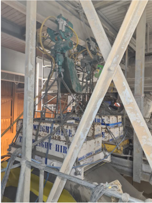
2 x 6t swl JDN air hoists in final monorail test position with test load.
