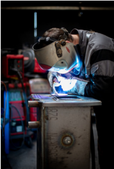
Figure 3: TransSteel Pulse in use at Guntamatic: The inner workings of the boilers are welded exclusively by hand.
