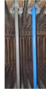
Fig. 10 – single tubes top coated with IGS 6003H and 6022
