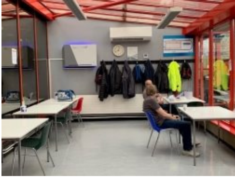
Soluva installation in Unit 161 canteen
