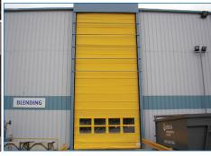
Roller shutter doors are offered single-skin or insulated. Finishes are galvanized, standard Plastisol or powder-coated to standard RAL or BS colours.
