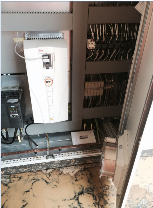
Caption: Replacing a fixed speed pump motor with one that is variable speed controlled has reduced pump failures and cut maintenance and energy costs
